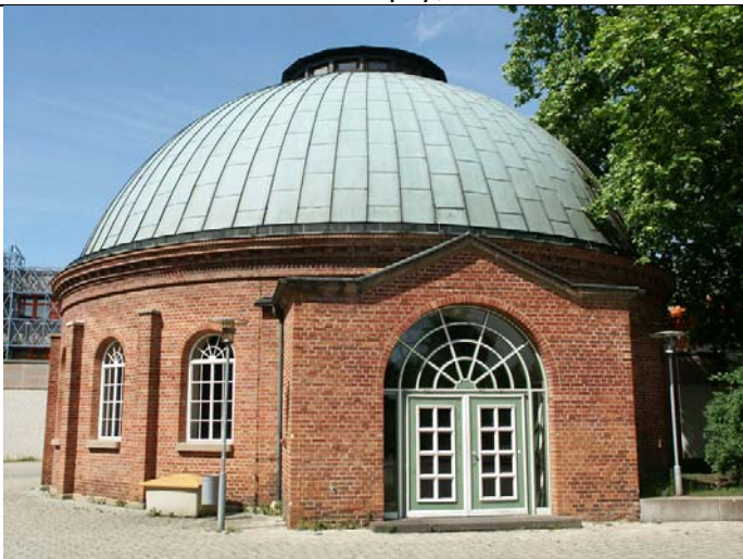
Giesshaus (casting house, seats 130)
